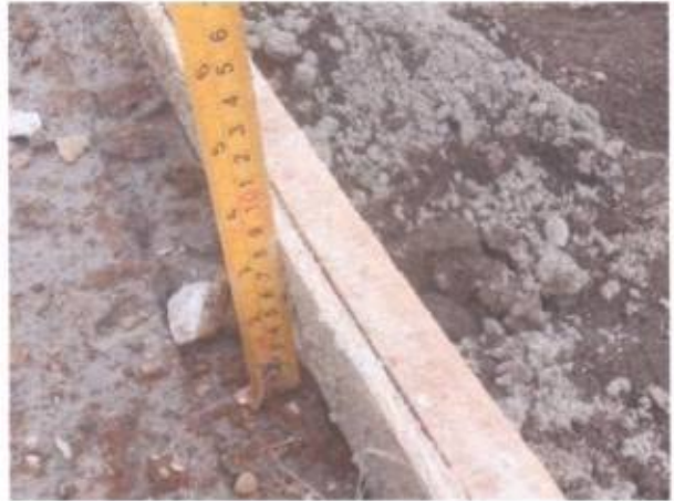
PEK. LANTAI BETON LANTAI FC' 10 MPA
