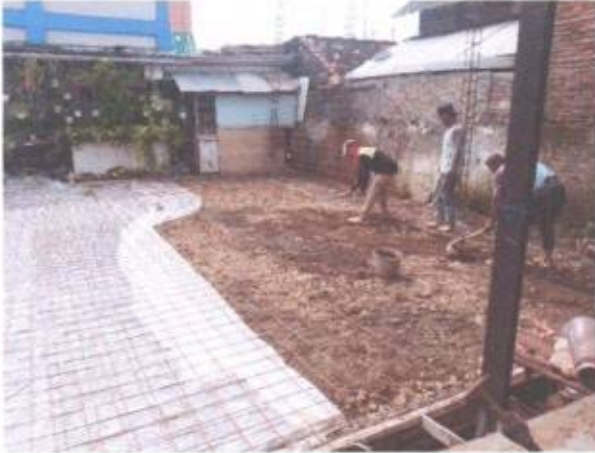
PEK. LANTAI BETON LANTAI FC' 10 MPA
